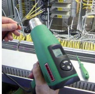
Shrinking of cable lettering
