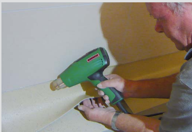
Rapid shaping of floor coverings
