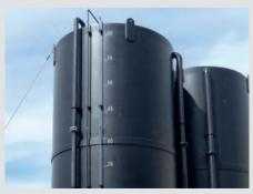
Storage tanks made of polyethylene
