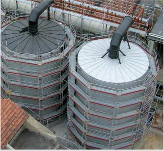
Air purification system, Spain. Material: HD-PE
