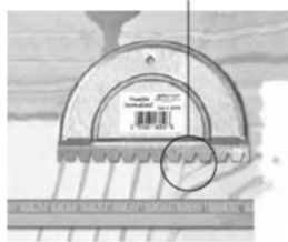
Example of properly troweled adhesive application
