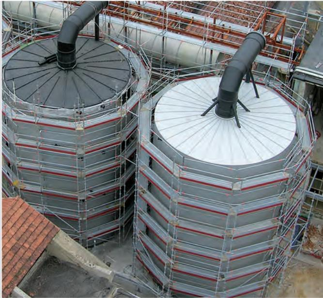
Air purification system, Spain. Material: HD-PE
